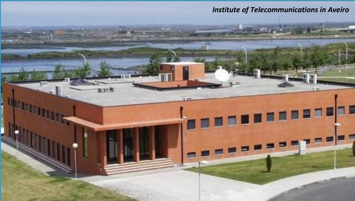
Aerial view of the Santiago Campus
